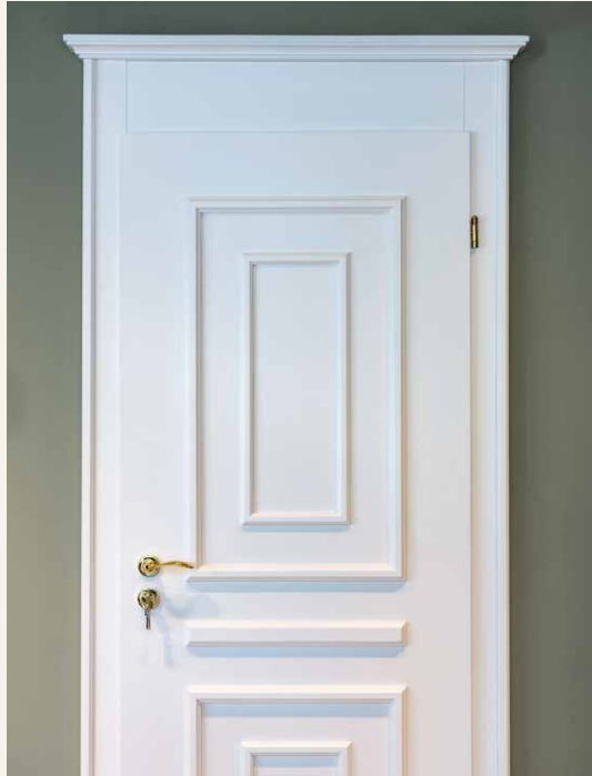
Door with wood moulding on door leaf and architrave
